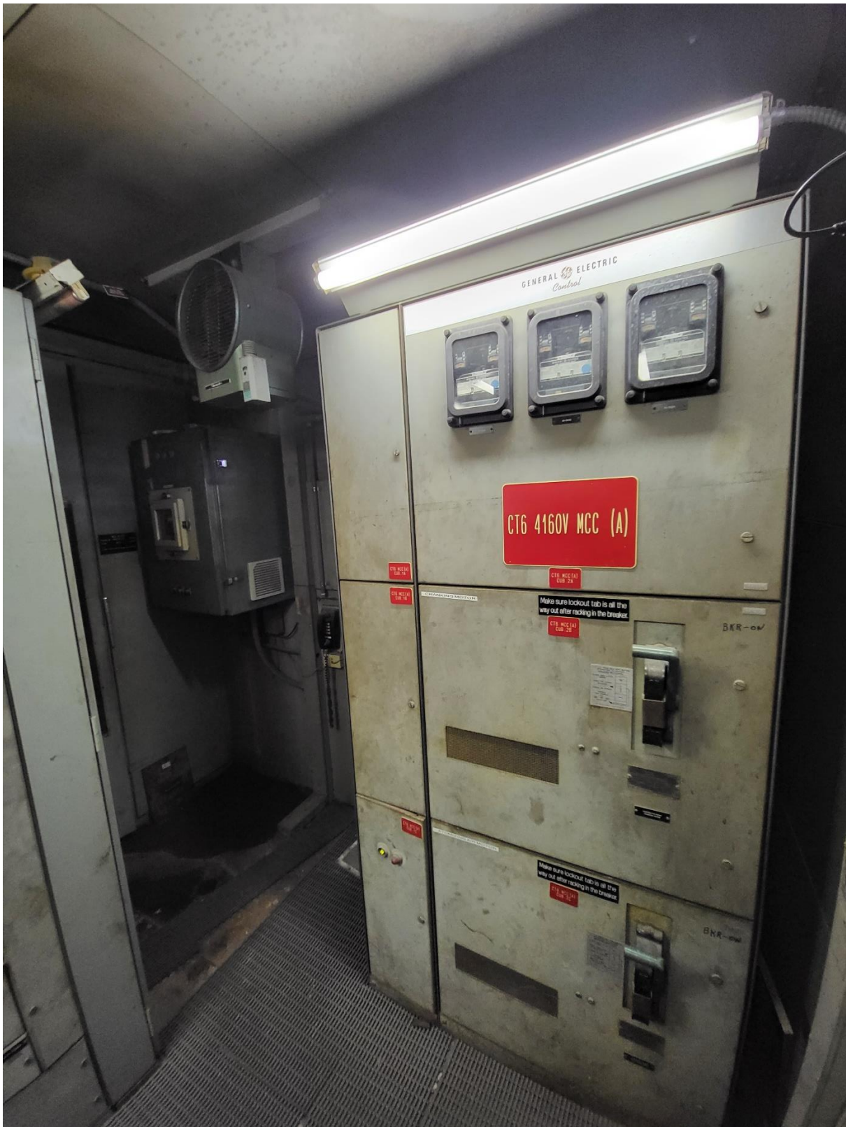
Current CT6 cab – southern half (showing MV MCC and heater)
